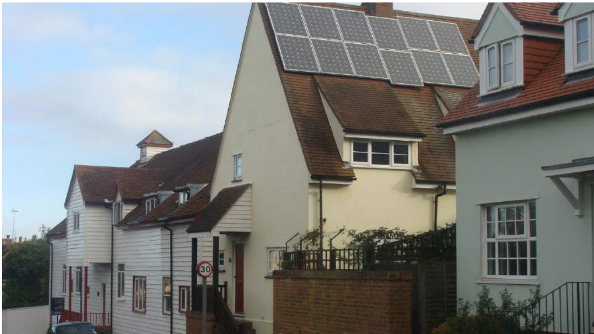
Picture 14. The impact of solar panels. This example is not in EHDC area where, to date, the impact of such equipment is limited. Controlling such installations so that where permitted they are at the rear of dwellings would protect the District's conservation areas.
