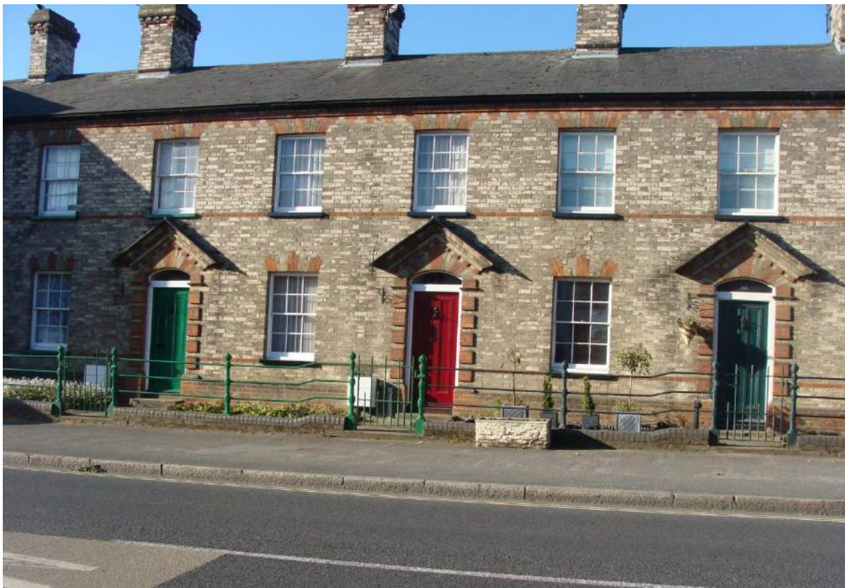
Picture 5. Co-ordination and visual integrity achieved by retaining original detailing. The successful character of historic terraces in part depends on simple repetitive detailing, including doors. Individual expression of ownership can be provided by painting doors different colours. (Not located in EHDC area).
