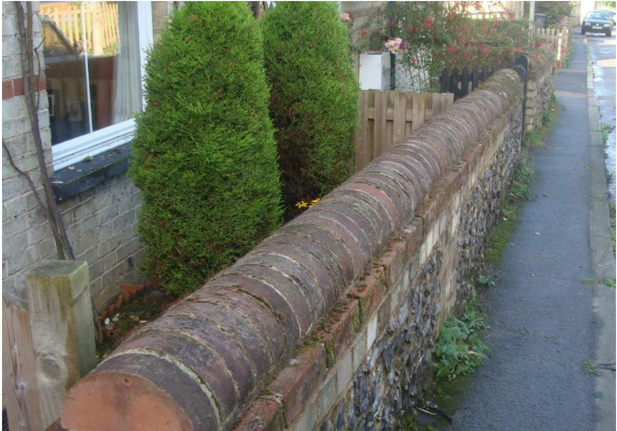
Picture 10. The demolition of a wall less than 1 m in height abutting a highway in a conservation area is not protected. Several such walls have been identified as candidates for Article 4 protection. Such walls below prescribed heights are in a minority.
